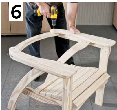
▲ With the chair bottom upright and the four legs firmly on level ground, the middle back rail is ready to be fastened to the armrests with bolts.
