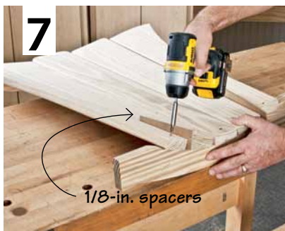
▲ When assembling the back, work from the center out and from the top down.
